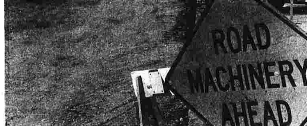
Reconstructing Legion Drive
